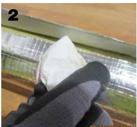
Before sealing, the mineral wool pipe section must be pressed together exactly. It is important to ensure that all adhesive points are free of dust, grease, and moisture before closing the adhesive tape!
