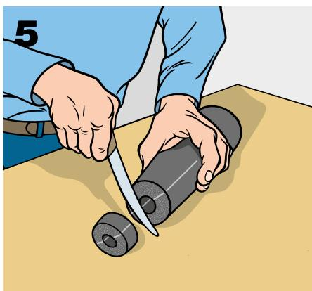
Take a piece of K-FLEX® the same diameter as the larger of the two pipes, and cut it slightly longer than the space left between the two sections of tubing already in place.
