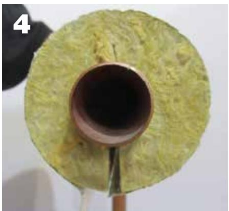
To minimize heat loss when installing horizontally, align the longitudinal seam so that it is at the bottom of the pipe! <sup>1)</sup>
