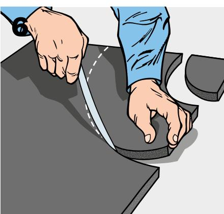
Place the section obtained on the reverse side of another sheet and use it as a template to cut out a second, mirror image section.
