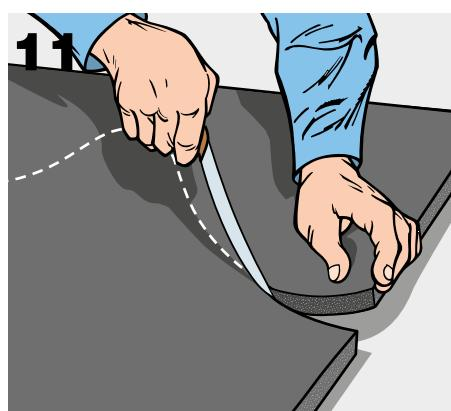
The cap should slide on and off easily. Once this is ensured, stick the edges together with K-FLEX® glue.
