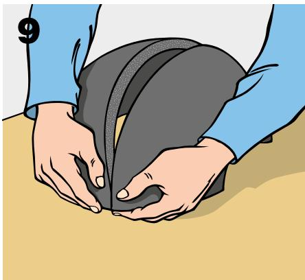
Wrap the K-FLEX® insulation around the pipe and press the edges tightly together.
