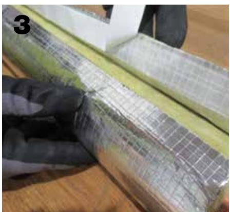
The longitudinal joint can then be sealed with the factory-fitted longitudinal overlap. Ensure the Adhesive overlap is pressed on well to ensure complete adhesion.
